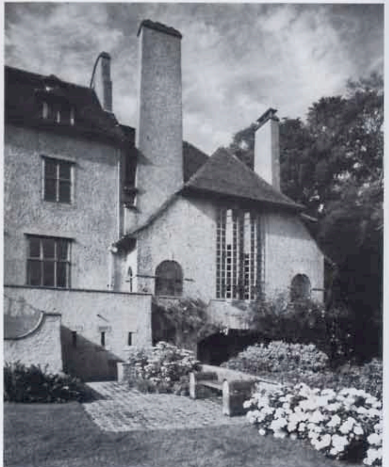
8—THE GARDEN FACADE OF THE LIVING HALL. The tall mullion window (with wooden mullions) is combined with two oriels
